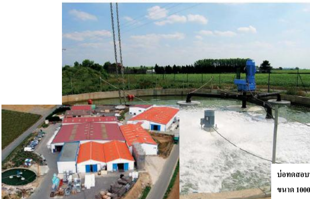
Concrete test tank - Volume 1000 m 3
